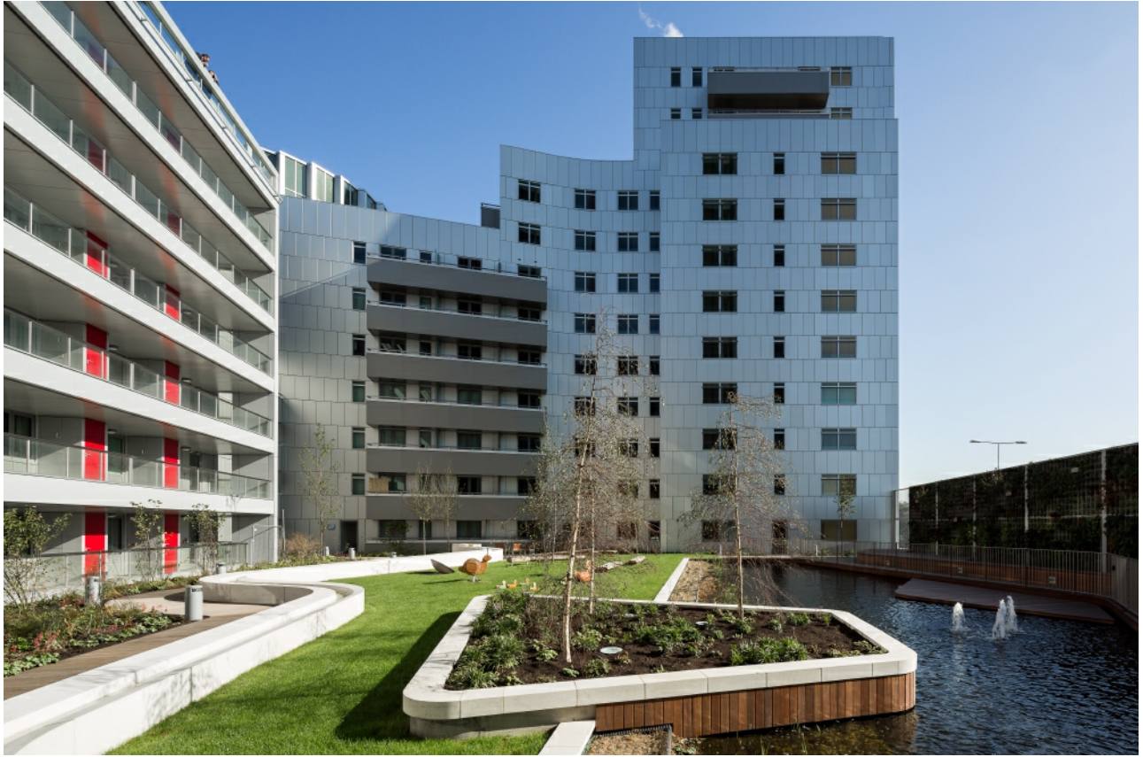
The buildings of the Vermillion phase are organized around a second-floor courtyard. Photo: © Tim Crocker
