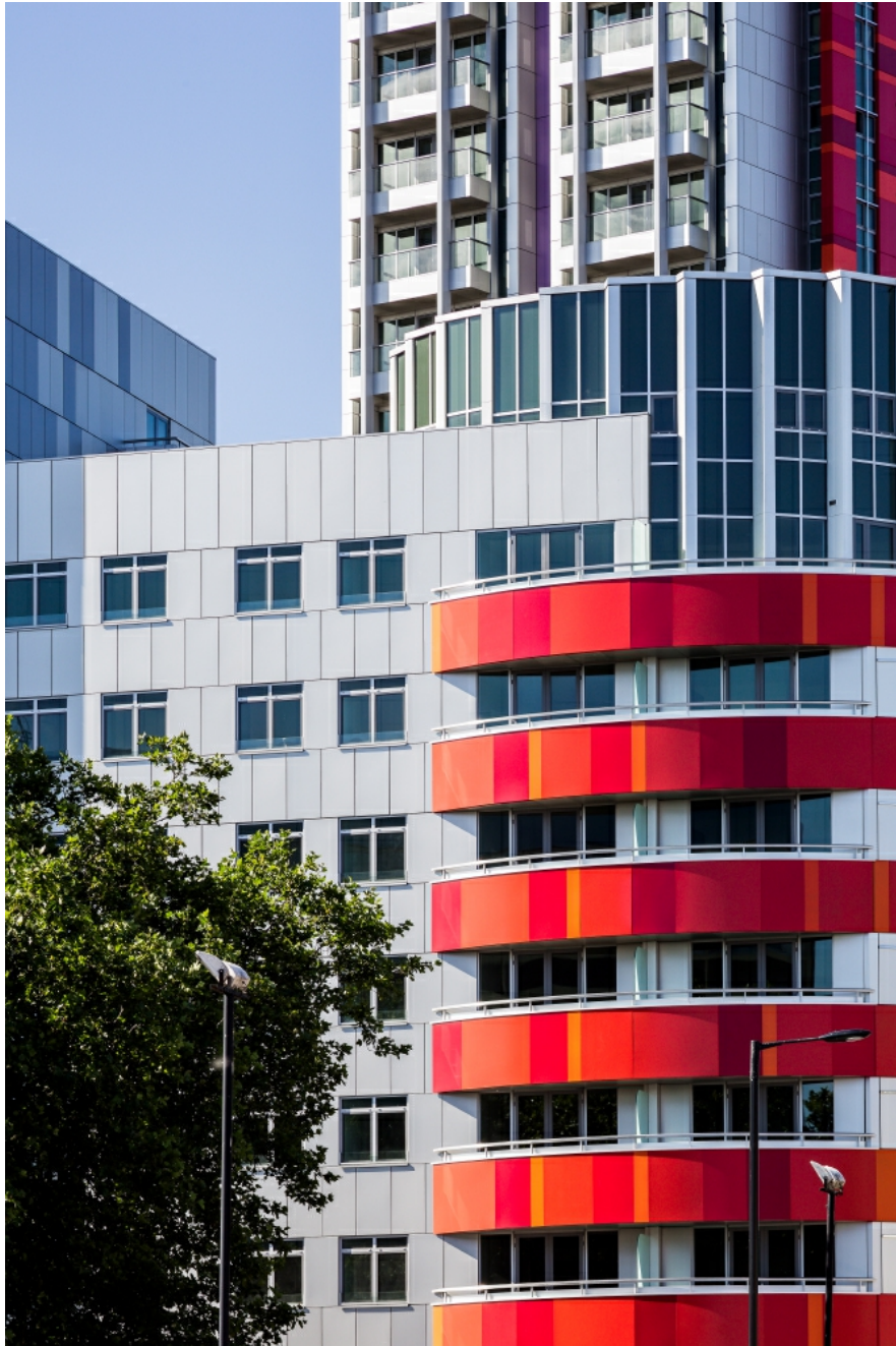
Facade detail. Photo: © Tim Crocker
